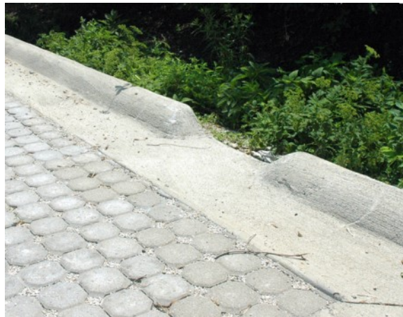
Figure 9.4-B: Cuts in the continuous curb allow for stormwater to be directed into landscaped areas.
