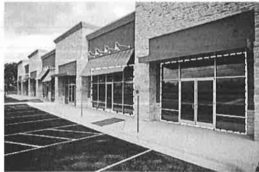
Figure 10.9-A: The window area is illustrated within the dashed line area for the two storefronts in the above image.
