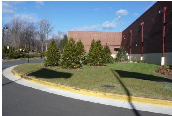
Figure D: The above image illustrates a vegetative screen that hides HVAC equipment and a dumpster.
